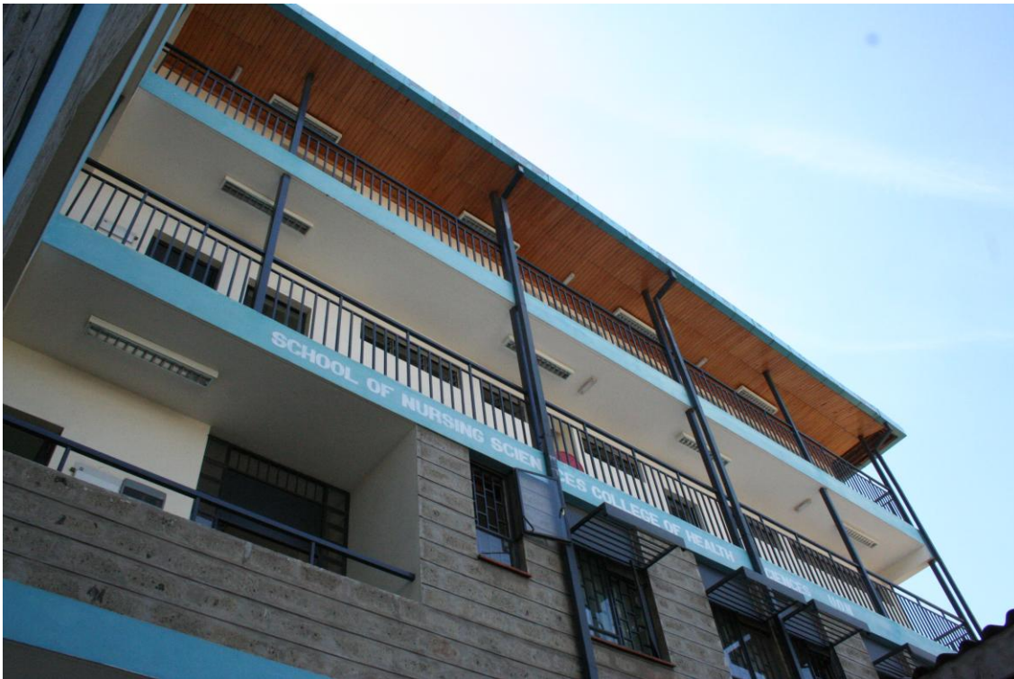
School of Nursing Sciences, College of health Sciences located at the Kenyatta National Hospital Campus
